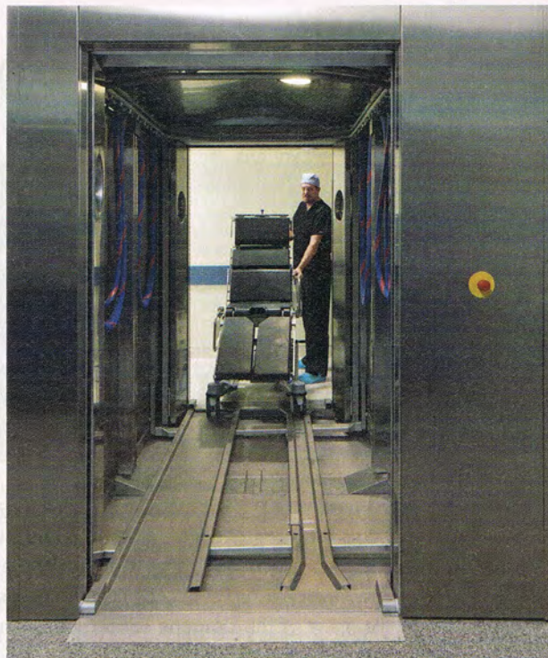
Renaissance Surgical Arts at Newport will utilize two discreet, low-intensity, stand alone sterilization areas between its operating theaters and a central high-intensity, processing area central to the operating corridor for main processes Photographer: Terrance Williams of Wundr Studio
